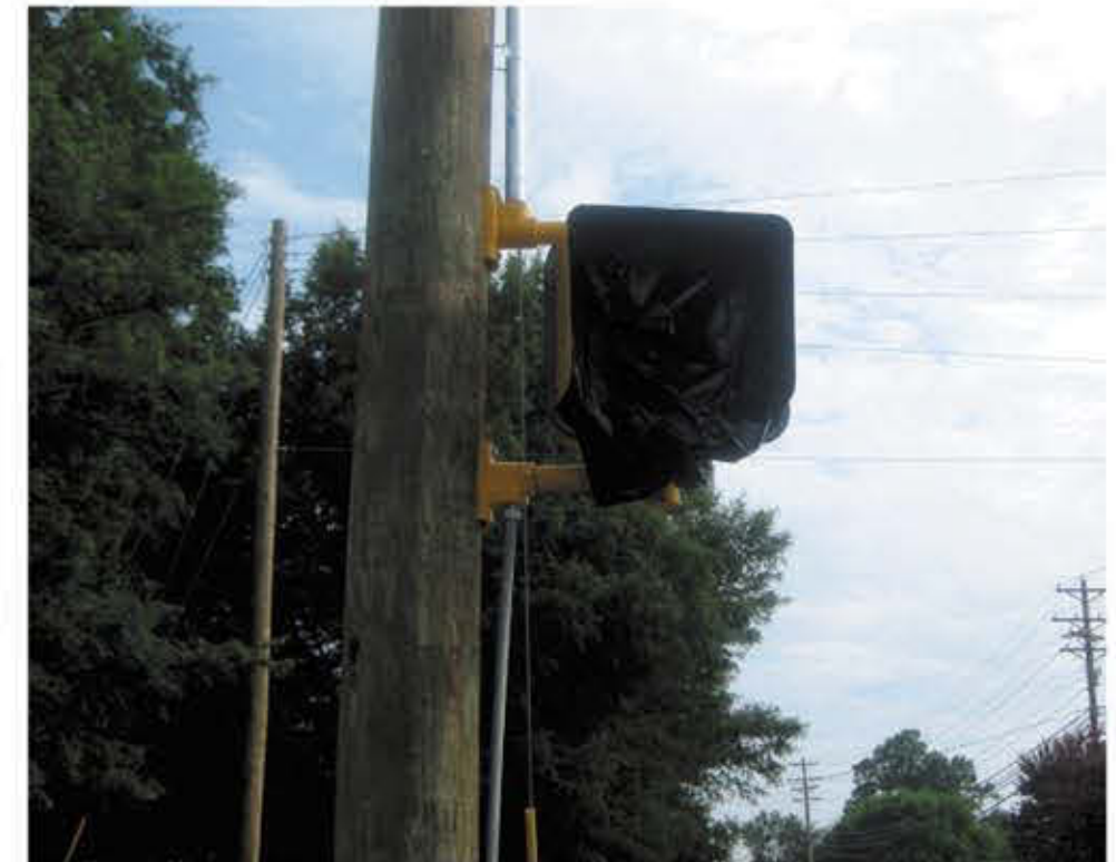
New walk/don't walk signs and push buttons were installed but not activated
